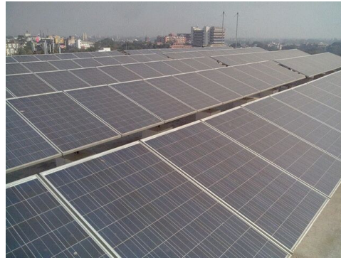
NMC – Main Bldg
